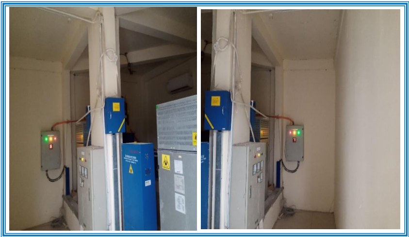
Area ruang mesin/rumah bed lift lt. rooftop
