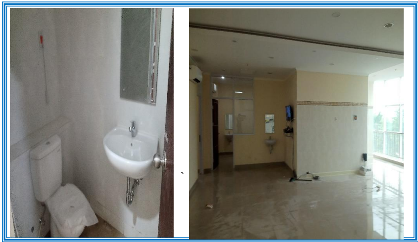
Closed, wastafel & area Ruang Nurse station Inst.HCU lt. 04
